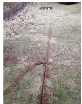
Trench dug by hand for water header
